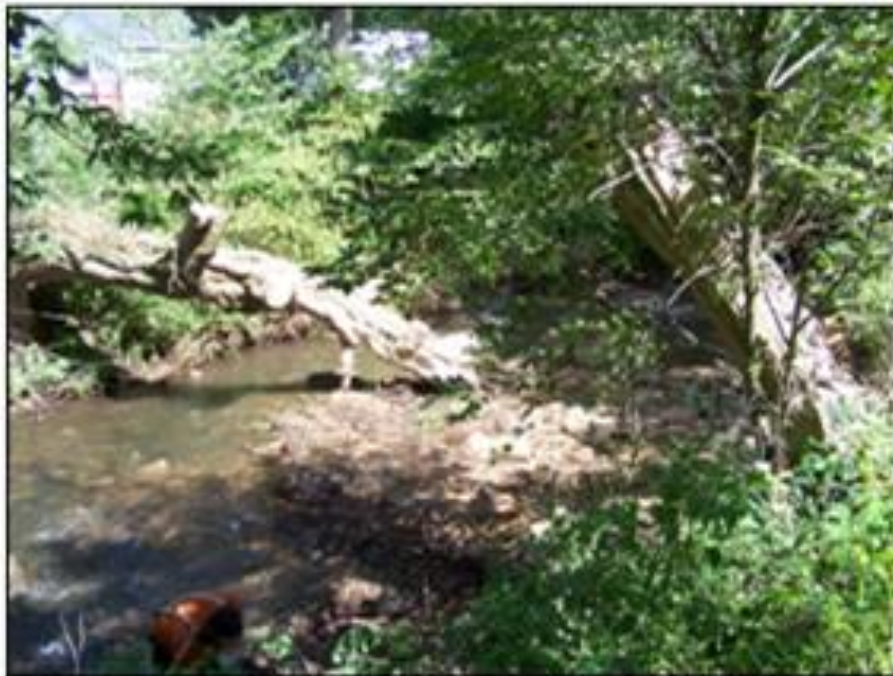
Figure 4: Completed logjam removal.
