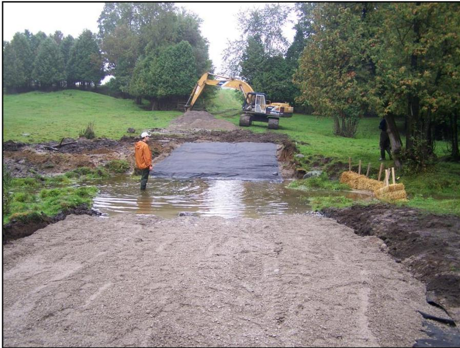
Figure 2: Laying Sand, geotextile and silt fencing down while re-creating stream crossing.
