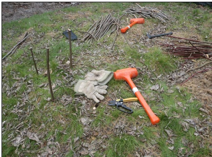
Figure 1: Live shrub staking.
