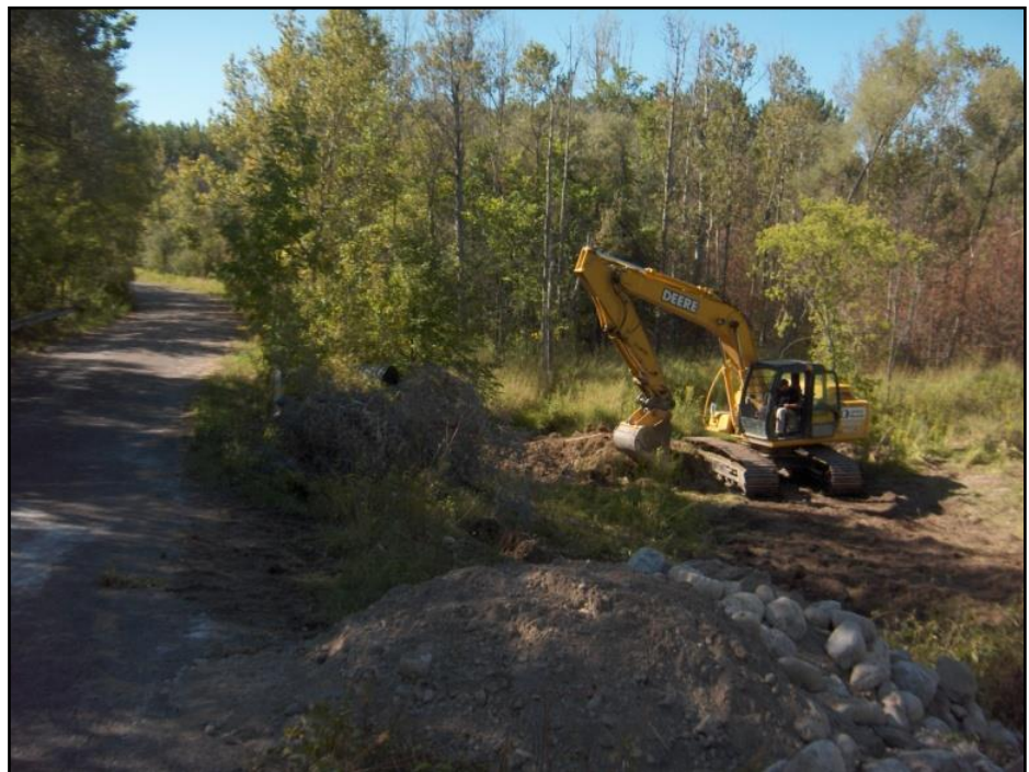
Figure 1: Contractor working on Gabion Basket Removal at Claremont Outdoor Education Centre.
