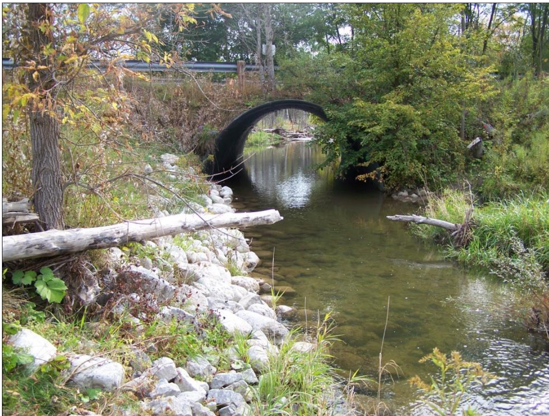
Figure 3: Bank enhancement site one year after restoration.
