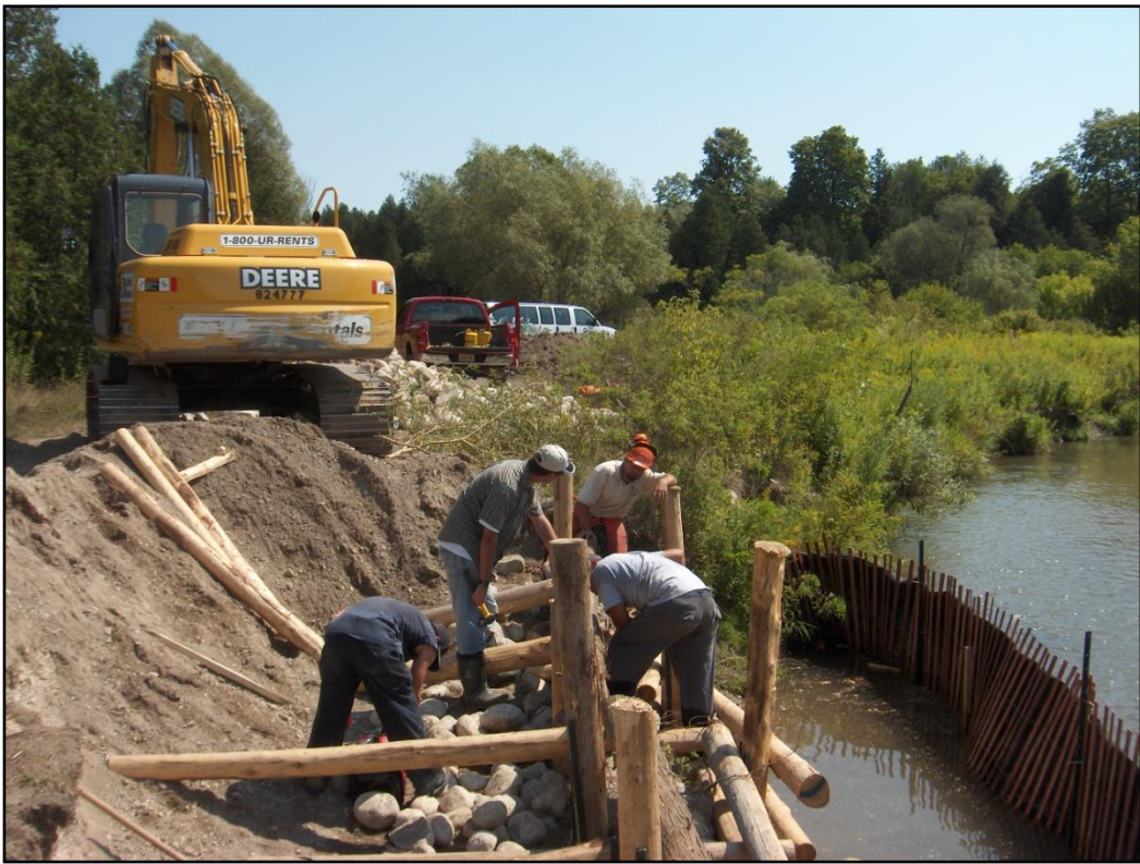
Figure 2: Staff installing the crib wall at Greenwood Conservation Area.
