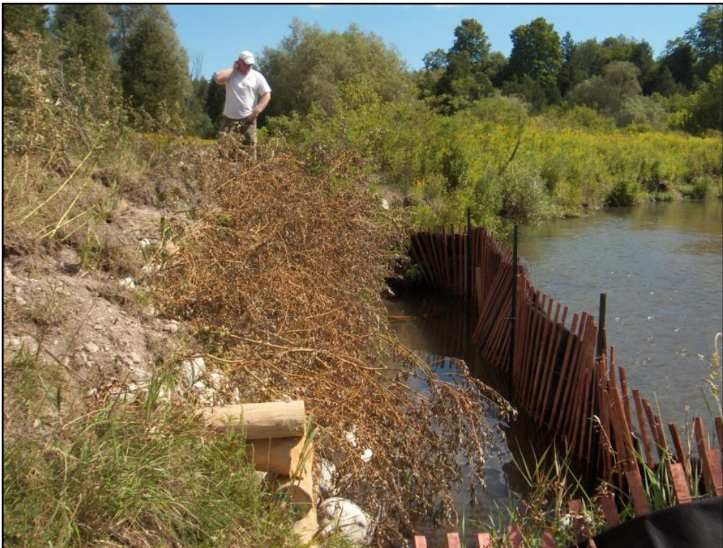
Figure 3: Upon completion an OFAH staff member surveys the live cribwall.
