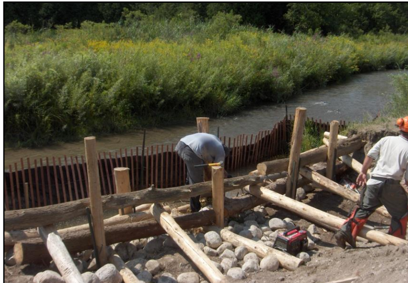
Figure 1: TRCA staff installing cribwall onto banks of creek.
