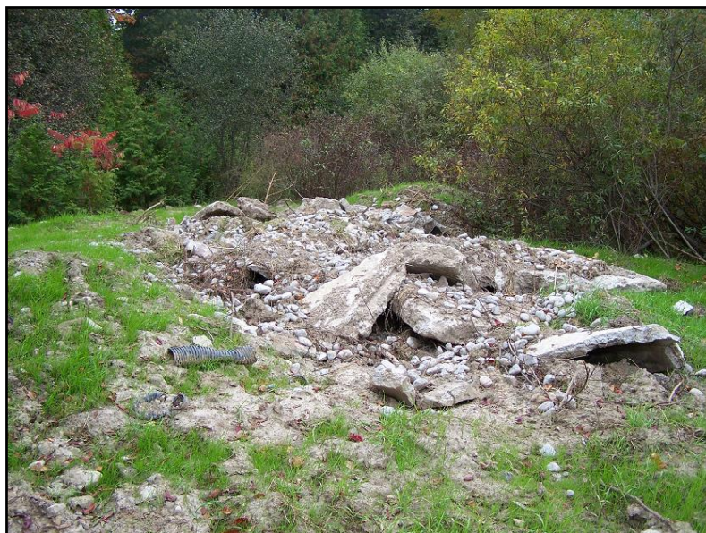
Figure 1: Snake Hibernacula created on golf course after cement bridge demolition.
