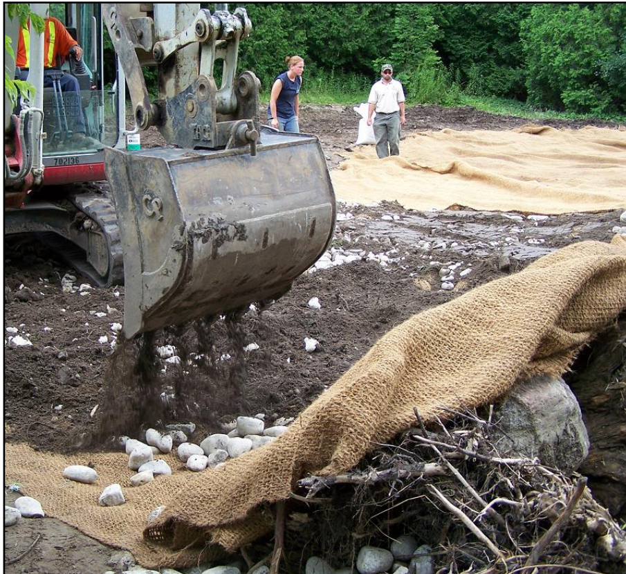
Figure 2: Core material was laid down and folded, additional localized soil and river stone were placed on top.
