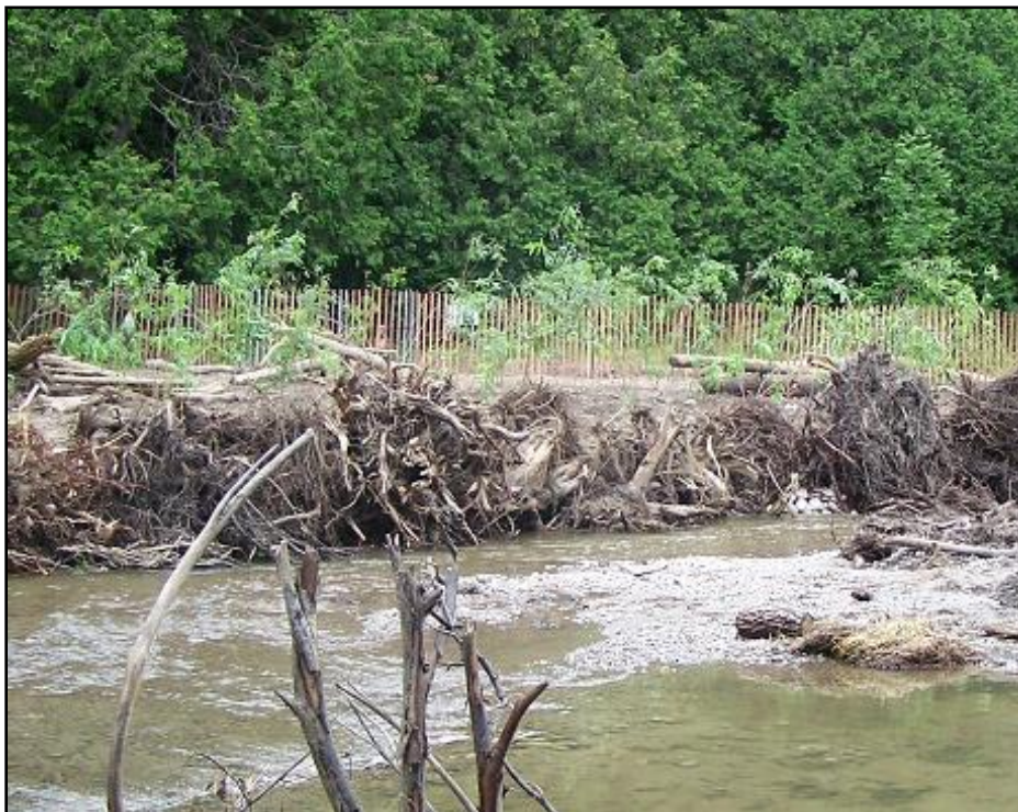
Figure 3: Completed bank stabilization project at Greenwood Conservation Area.
