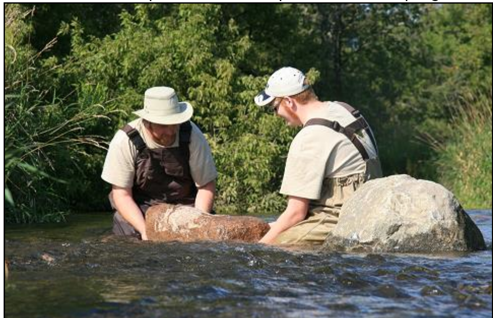
Figure 1: Placing boulders in the Cobourg Brook on the Holmes property to improve fish spawning habitat and resting areas.
