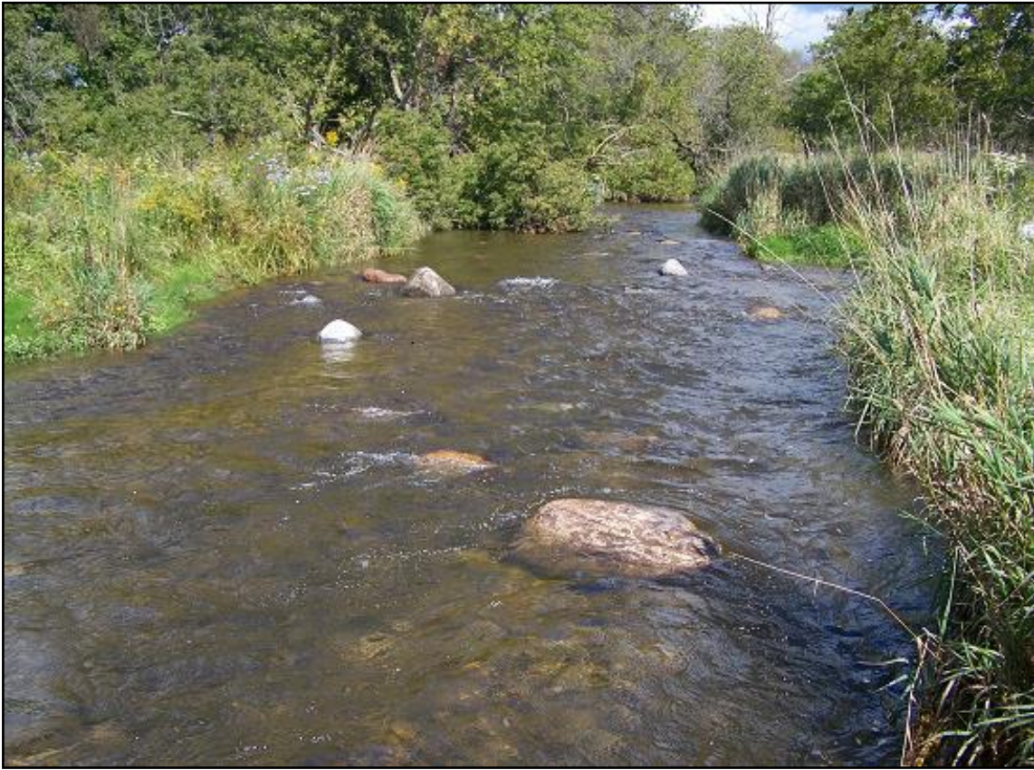
Figure 2: Completed boulder placement in the stream on the Holmes property.
