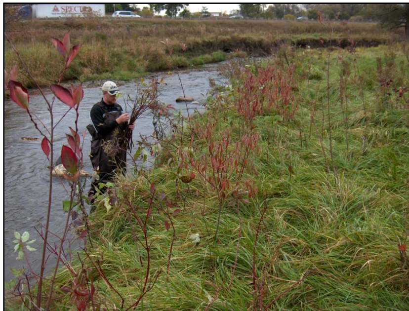
Figure 3: OFAH staff live staking of dogwood along Cobourg Brook.
