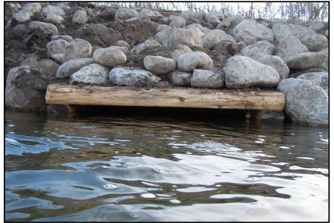
**Figure 3:** LUNKERS with boulders holding it in place in Cobourg Brook.
