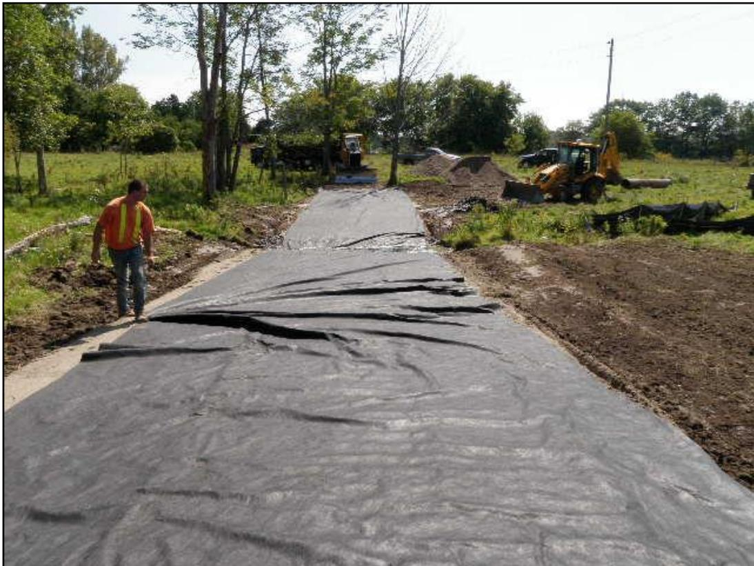
Figure 3: Placing synthetic cloth down to protect soil from washing away.
