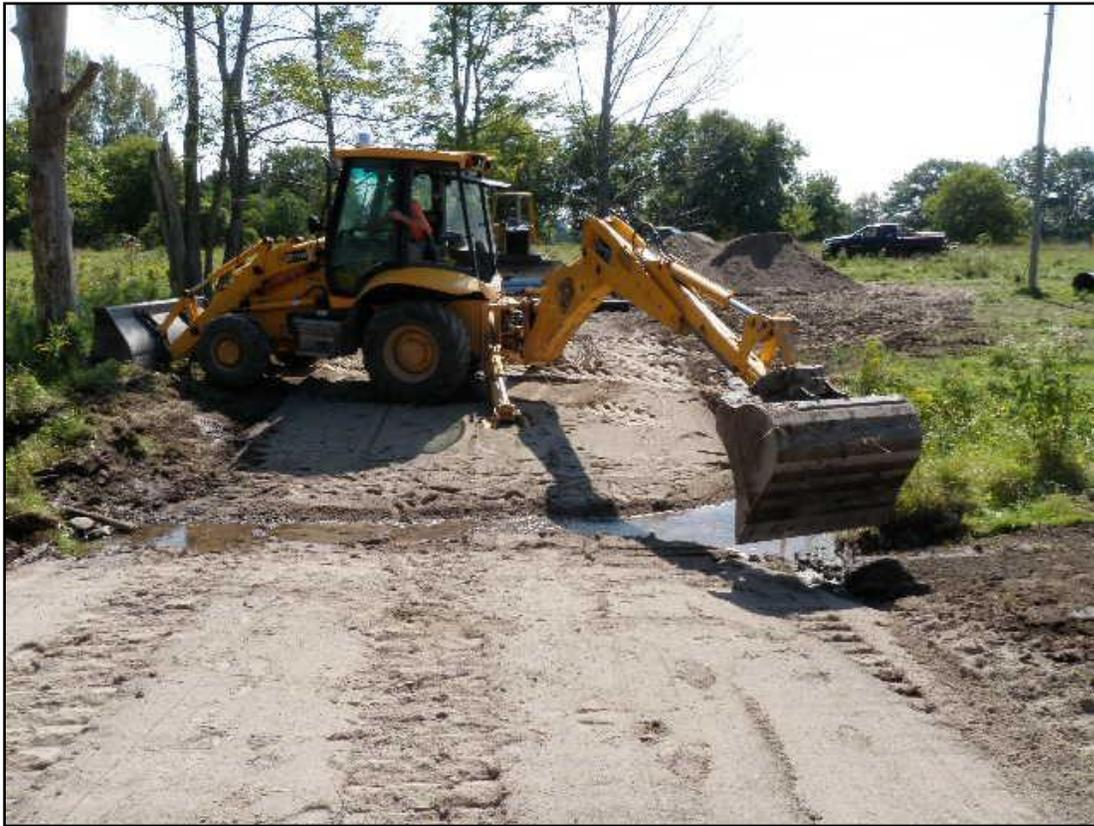
Figure 2: Re-grading of stream to bring slope to 8:1 ratio.
