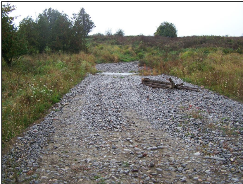
Figure 1: Low -level crossing created in 2007 on Barkey Property.
