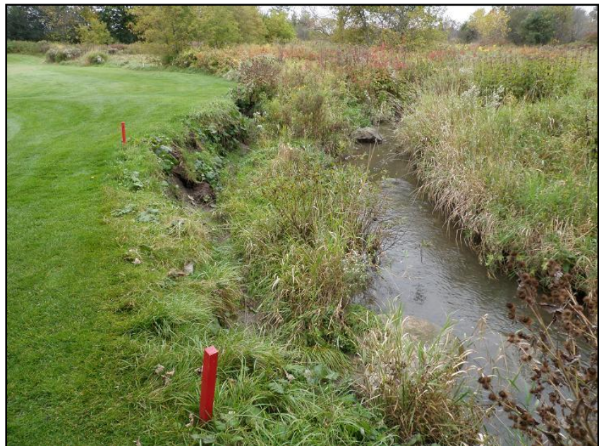
Figure 1: Stream bank of Duffins Creek on Bushwood Golf course, eroded and washing away into stream (before planting).
