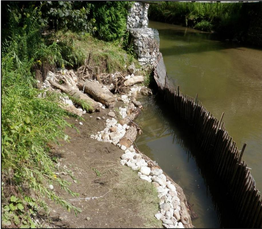
Figure 2: Root wads, logs and river stone in place along the bank to stabilize slope.
