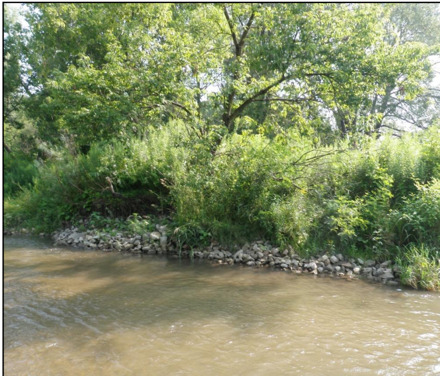
Figure 3: The completed stream restoration project with the river stone spread across 7m of the shoreline.
