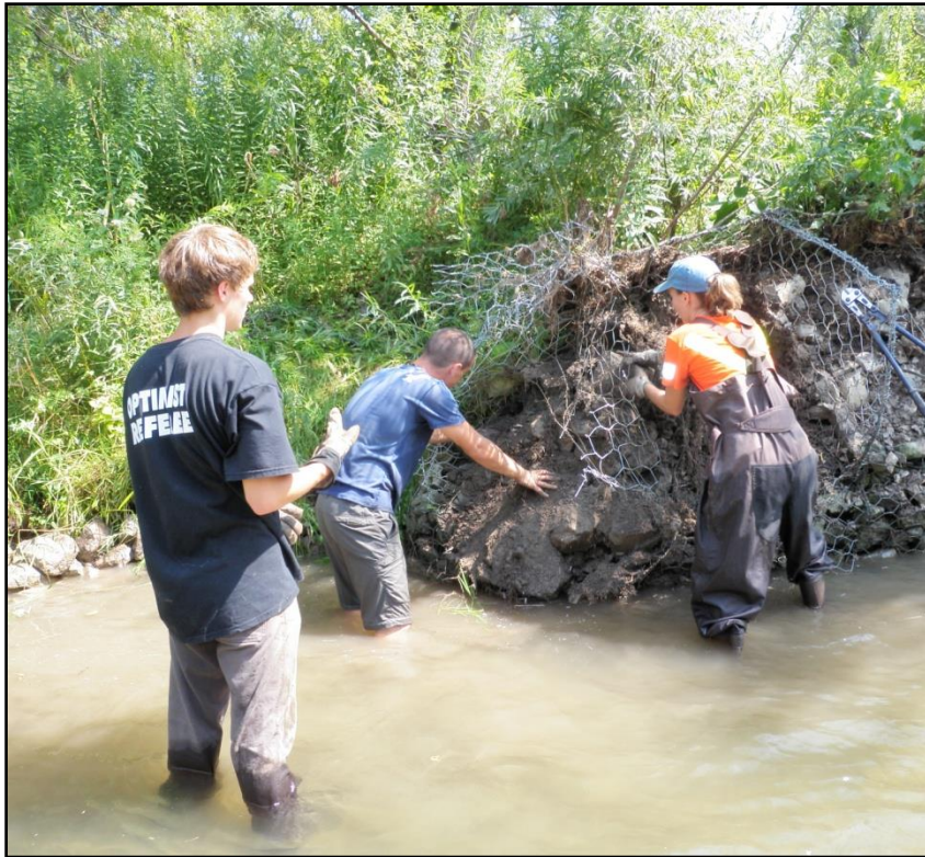
Figure 2: Volunteers disassemble and redistribute the gabion basket materials to other areas along the stream.
