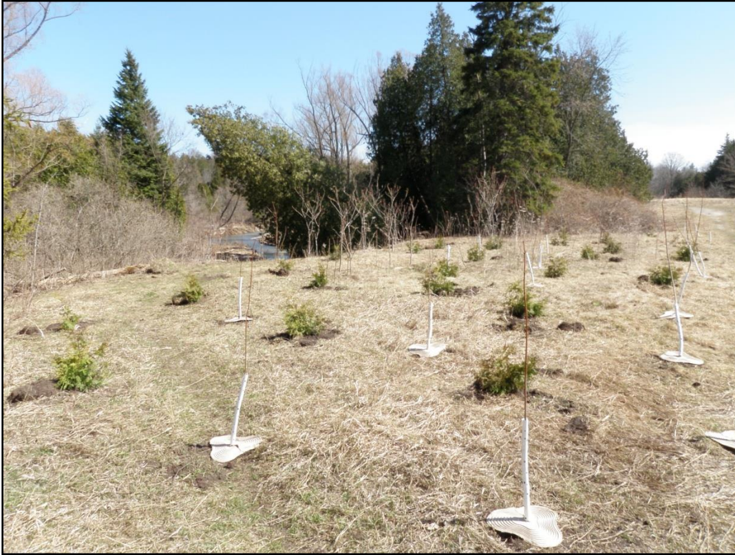
Figure 2: Completed planting of trees and shrubs along Duffins Creek to improve bank stabilization and water quality.
