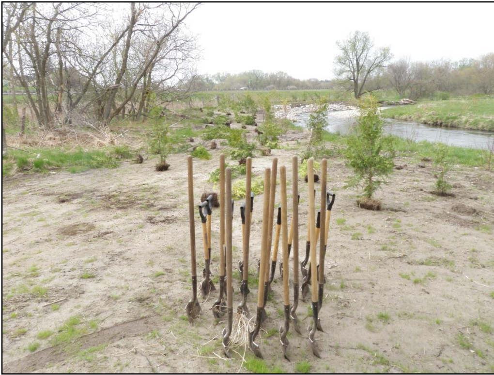
Figure 2: Materials for planting shrubs along the Cobourg Brook bank.
