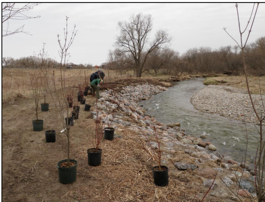
Figure 1: Site of previous bank stabilization project in 2008, the stream bank on the Holmes property is now being planted with trees and shrubs in 2009.
