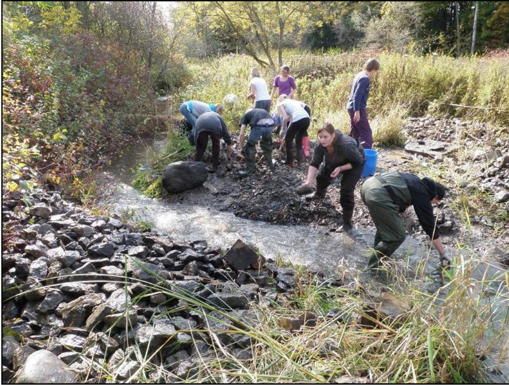
**Figure 2:** Port Hope High School students remove gabion by hand to restore flow of stream for fish passage.
