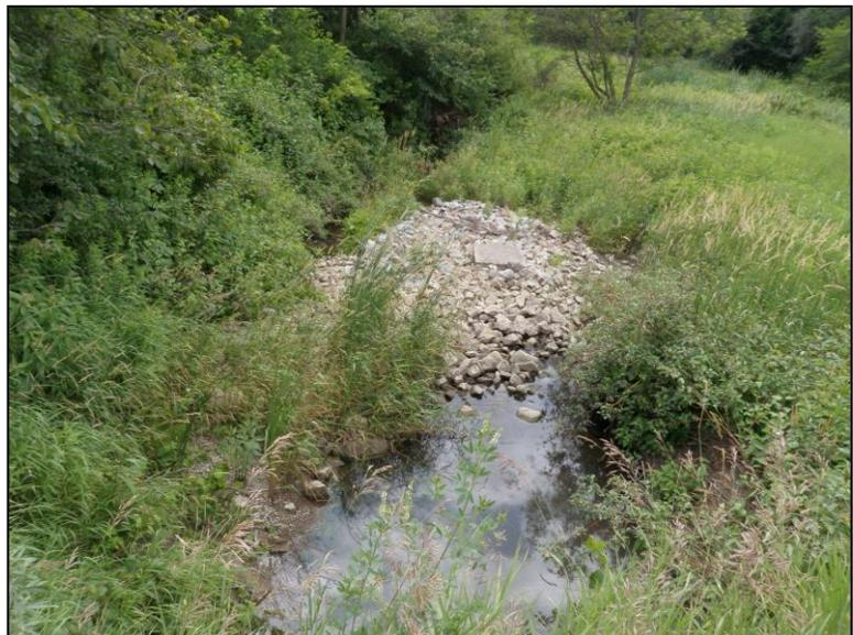
Figure 1: Failed gabion along Duffins Creek on the Transport Canada Lands in Pickering, Ontario.
