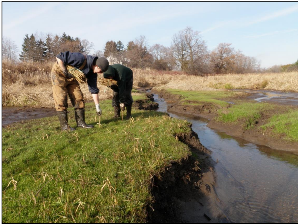
Figure 2: Planting live staked willows into the ground to stabilize soil.
