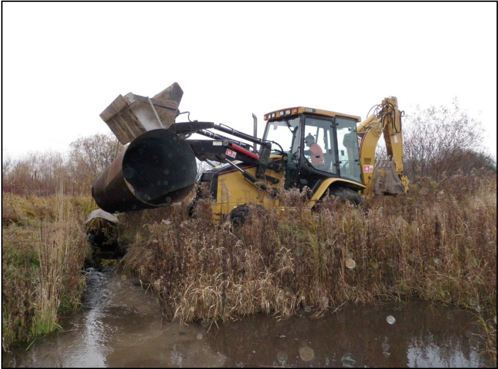
Figure 2: Culvert being removed on Transport Canada Lands property in Pickering, Ontario.
