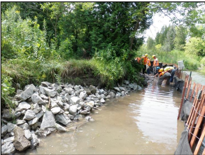
Figure 4: Staff members relocating stones along banks of Duffins Creek.
