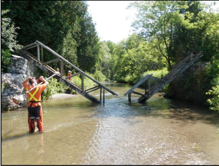
Figure 2: TRCA staff cutting down footbridge.
