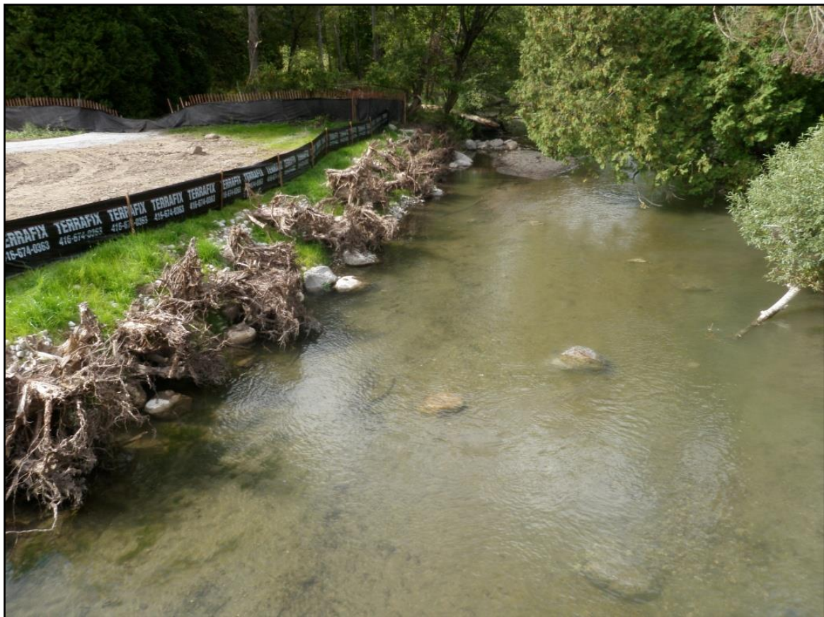
Figure 3: Boulders placed along the creek bottom in pods (groups of 3-5).
