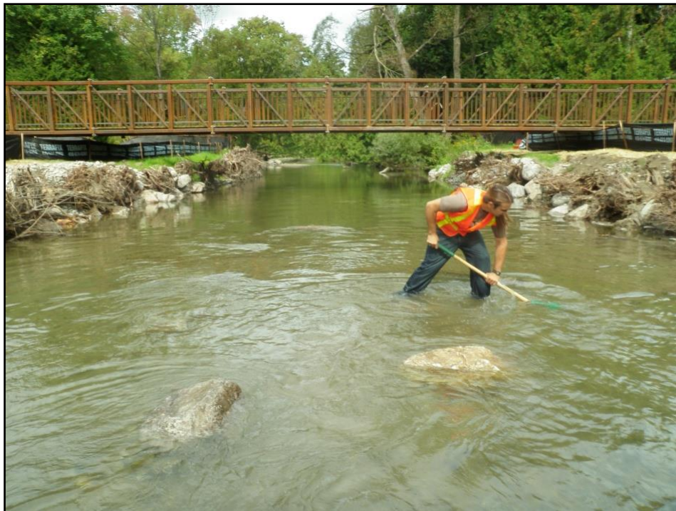
Figure 1: OFAH crew placing the boulders in the stream.
