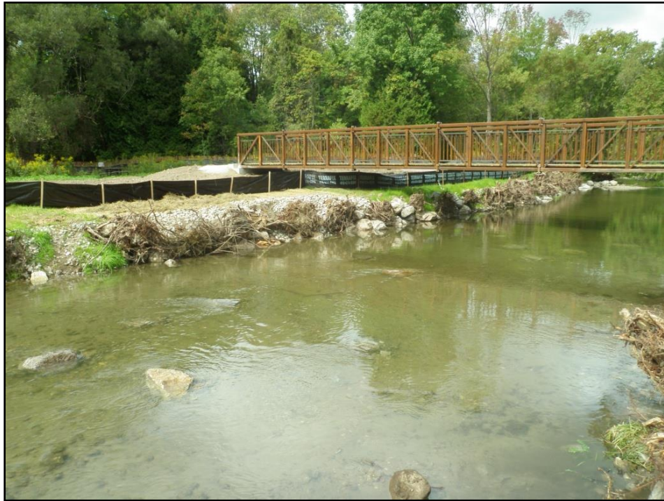
Figure 2: Finished boulder placement.
