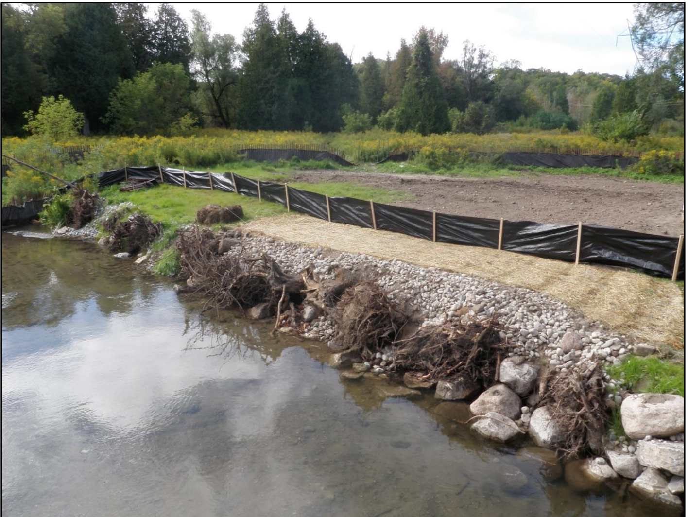
Figure 4: Completed root wad and bank stabilization project at Greenwood Conservation Area along Duffins Creek.
