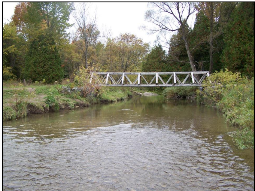
Figure 1: Before stabilization project began at Greenwood Conservation Area in Pickering, ON.
