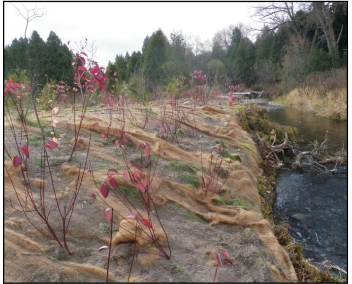
Figure 3: Completed planting on the Hie property in Cobourg, Ontario.
