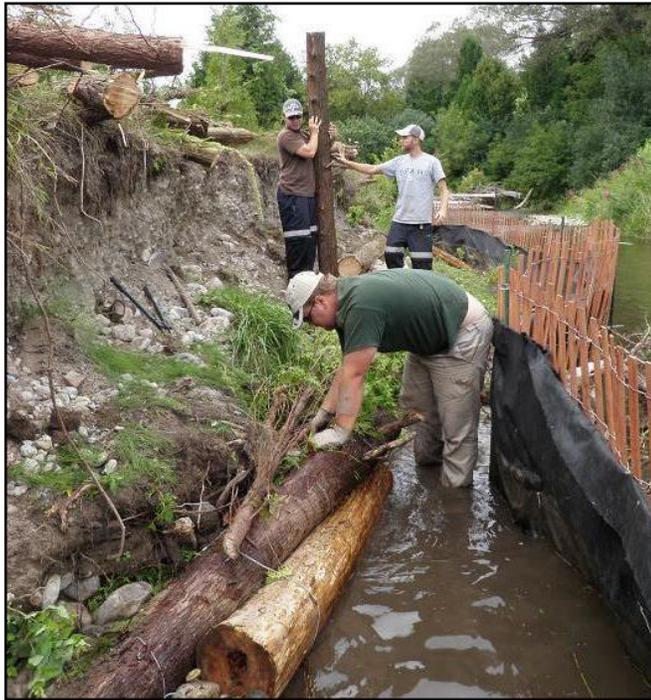
Figure 2: Installing logs and root wads to hold the bank in place.
