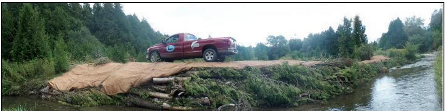
Figure 4: Completed project - 60m of bank stabilization.
