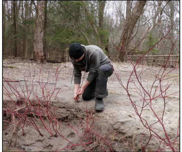
Figure 3: Volunteer placing live red osier dogwood stakes into the stream bank for stabilization.
