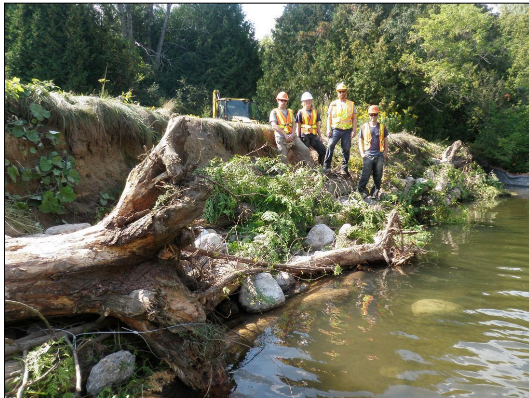
Figure 3: Completed revetment project with the TRCA crew standing on the root wads.
