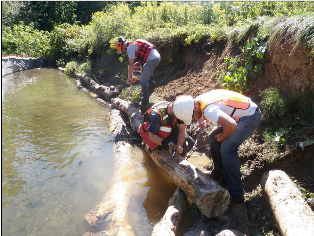
Figure 2: MNR and TRCA crew anchoring root wads along the stream bank with aircraft cable and soil spikes.
