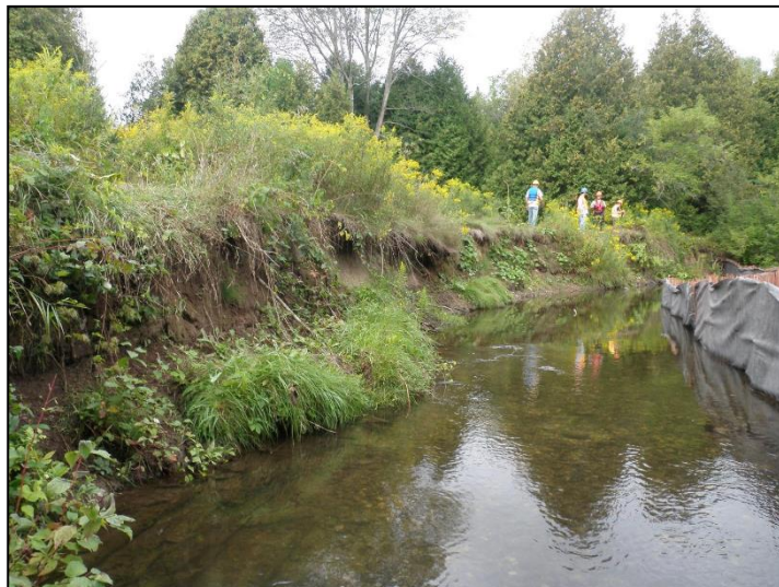
Figure 1: Revetment site before restoration with eroded banks.
