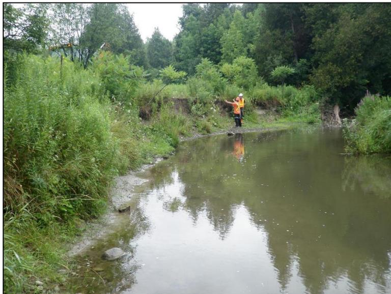
Figure 1: Revetment site before restoration with eroded banks.
