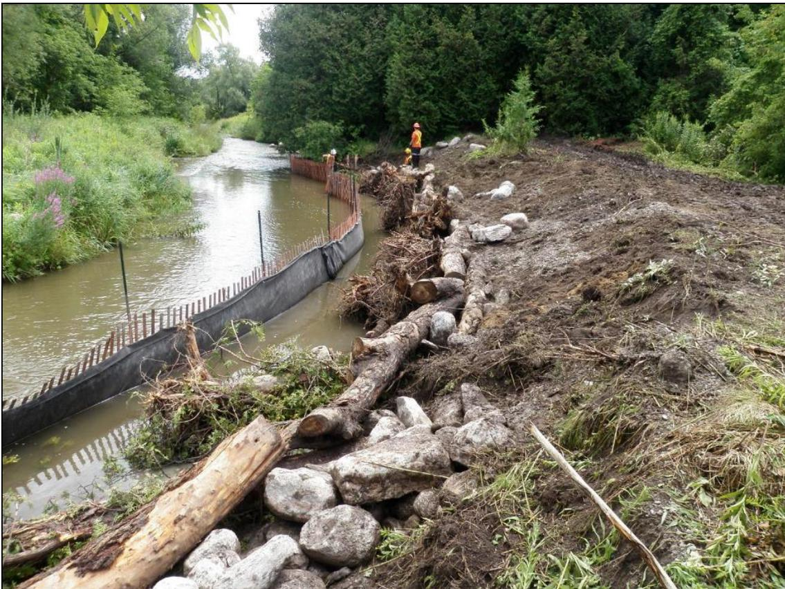
Figure 3: Revetment site downstream photo nearly completed.
