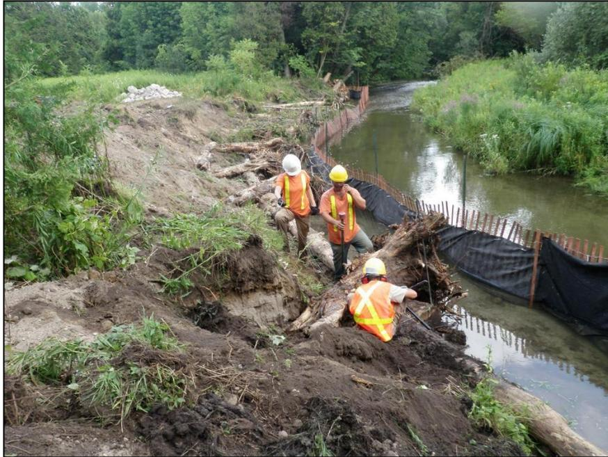
Figure 2: OFAH and TRCA crews anchoring root wads along the stream bank.
