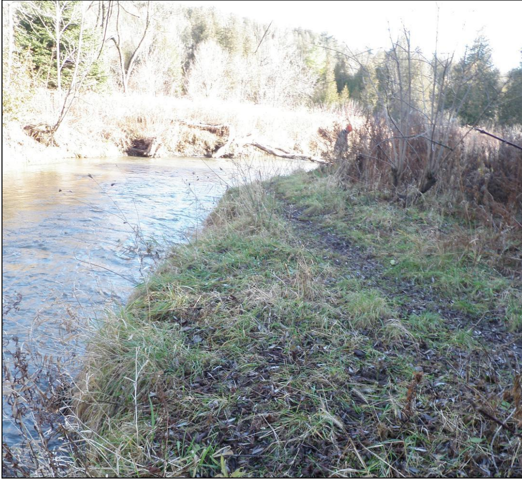
Figure 2: Bottom end of the project site, the stakes are not visible because they are pounded below ground to prevent frost heaving in the spring.
