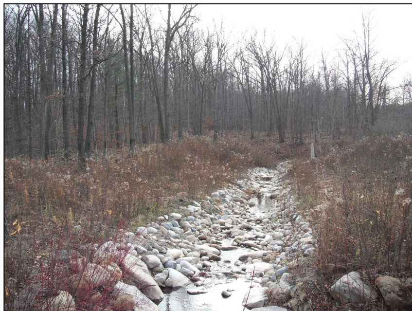
Figure 1: The channel downstream of the culvert before planting.
