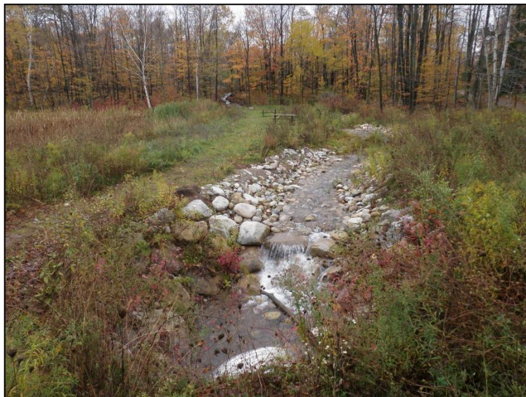
Figure 1: The bypass channel berm before planting, Wolfe Lake to the left.
