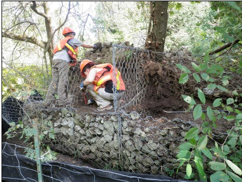
**Figure 2:** Ontario Stream staff and University of Toronto student volunteer cutting the wire basket open and removing gabion stone by hand.
