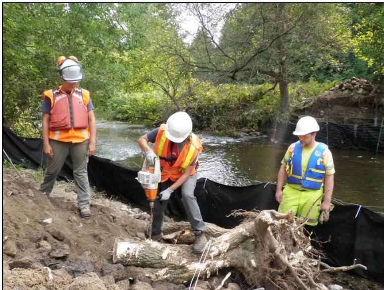
**Figure 3:** TRCA and OFAH staff installing a root wad in the stream bank.
