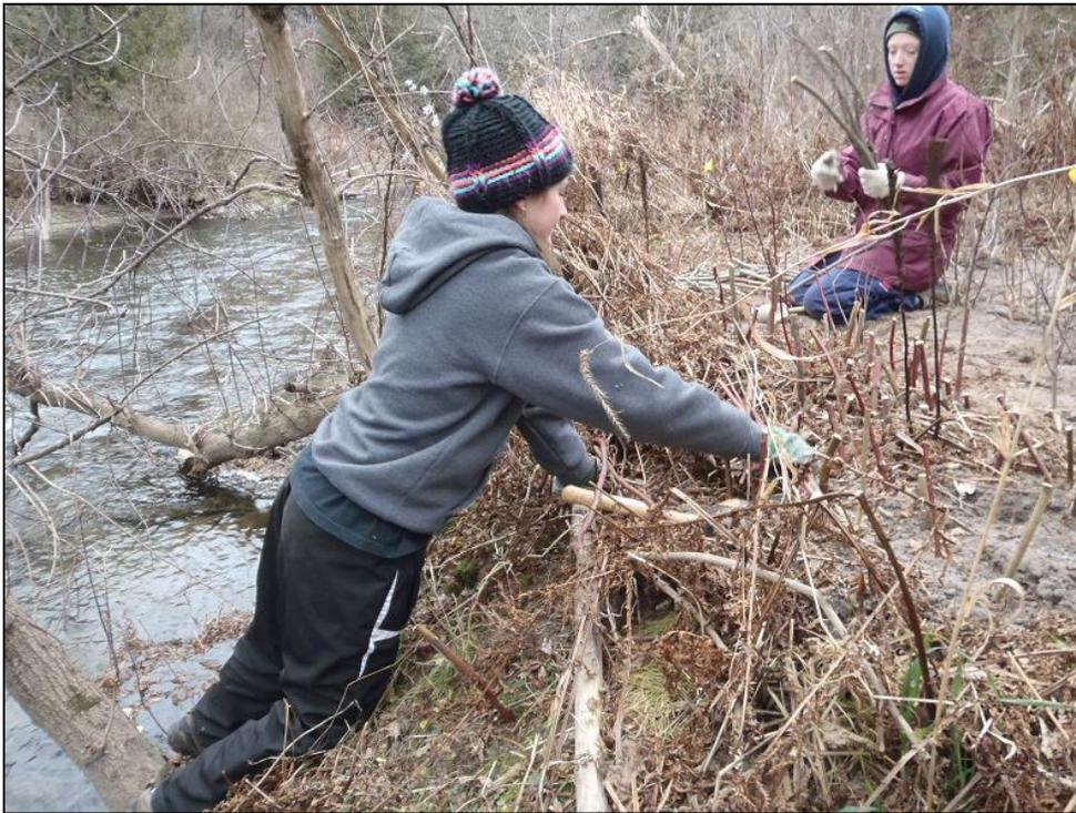
Figure 3: Thomas A. Stewart Co-op students installing live stakes along the stream bank.
