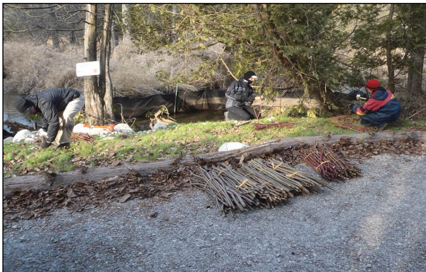
Figure 1: The revetment site at the start of the live staking.
