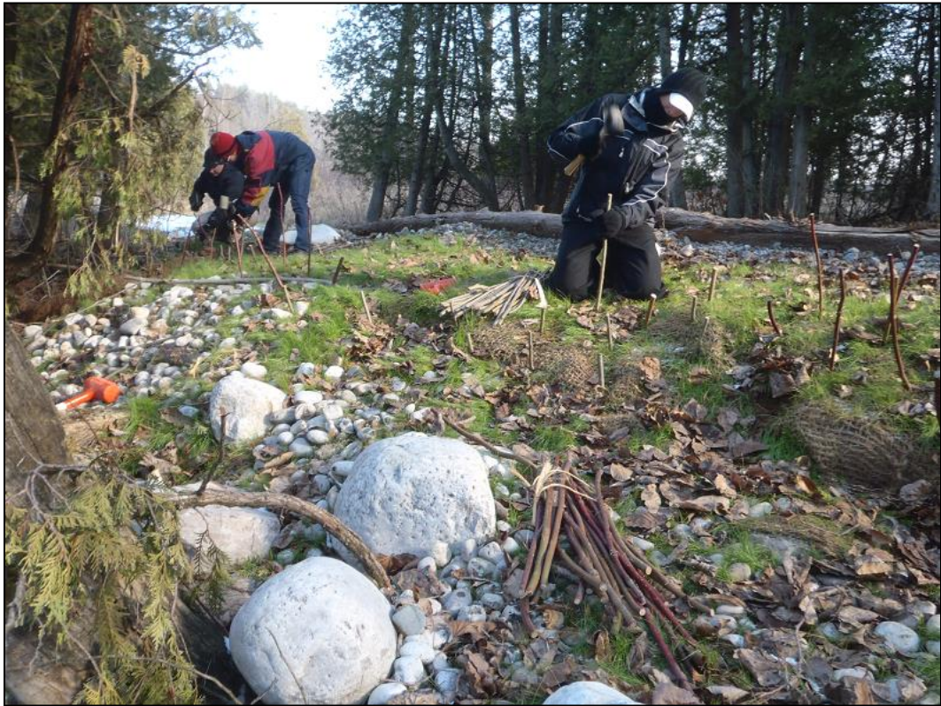
Figure 3: The crew inserting and hammering in the stakes with a mallet.
