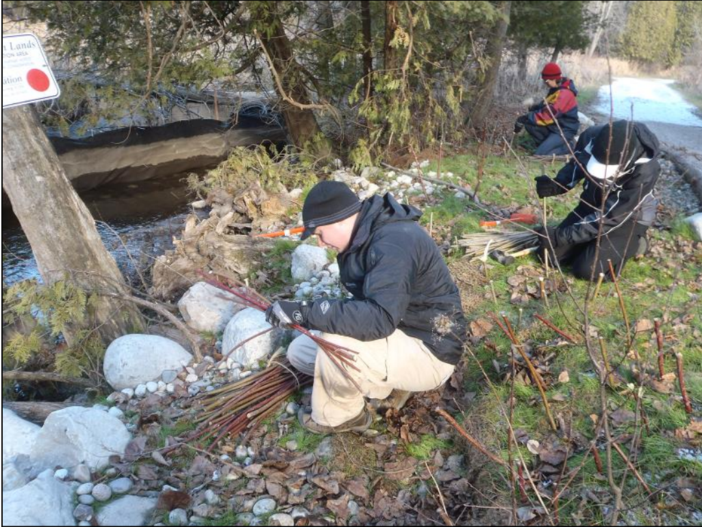
Figure 2: Live willow stakes being installed by Ontario Streams.
