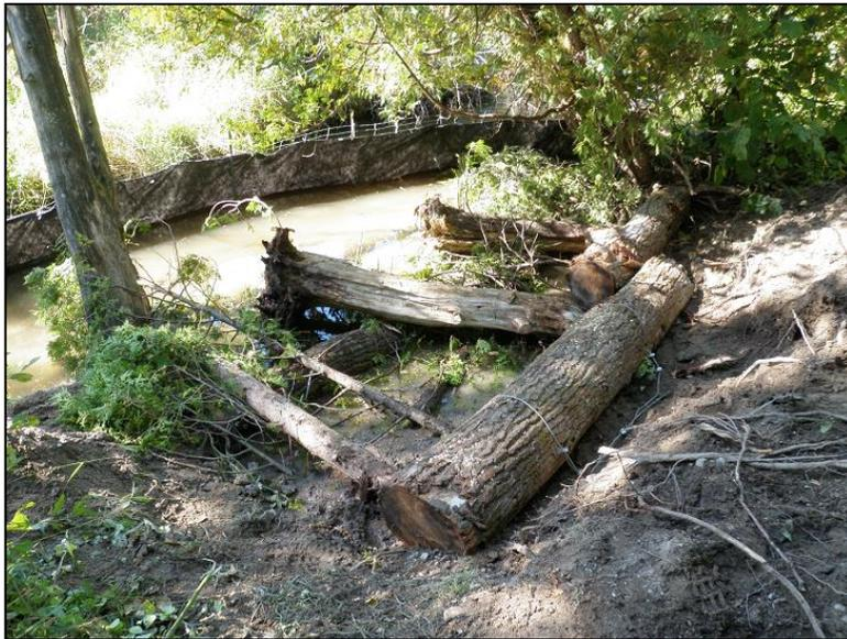
**Figure 3:** Revetment site before filling in the holes with stone and soil.
