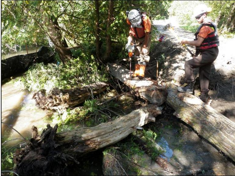
**Figure 2:** TRCA crew anchoring root wads along the stream bank.
