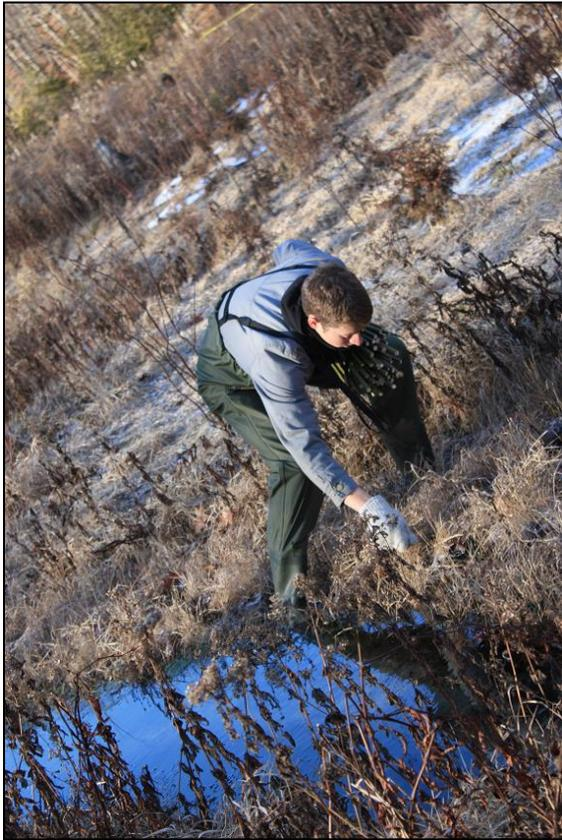
**Figure 2:** Student with a bundle of live stakes at the edge of the new channel.
