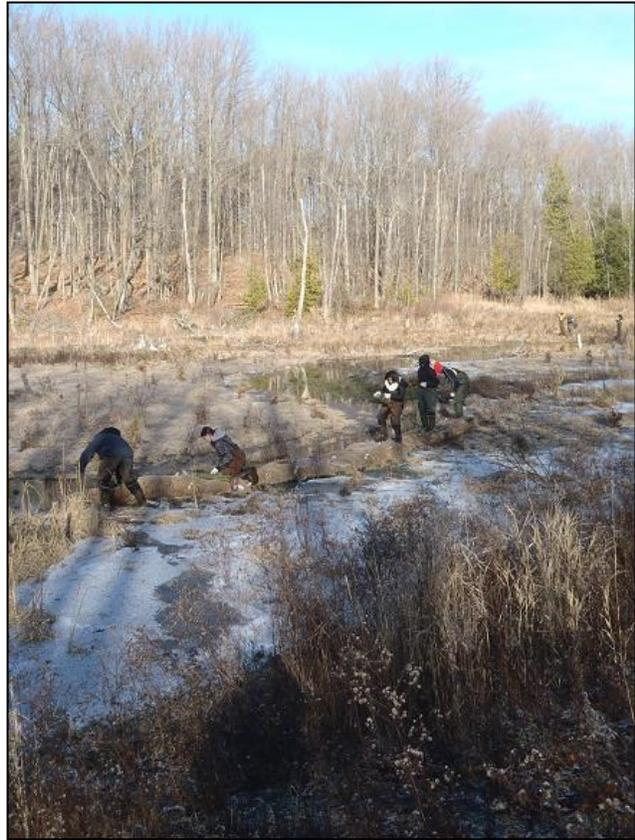
**Figure 3:** Student staking the outside bends of the new channel.
