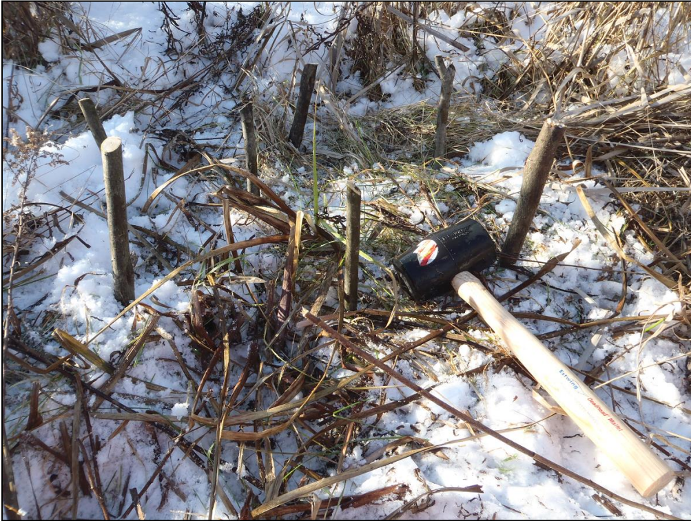
Figure 2: Mallet and seven live willow stakes partially inserted into the ground. The stakes are inserted below the layer of grass and soil is hammered overtop to prevent the frost from pushing them out of the ground in the spring.
