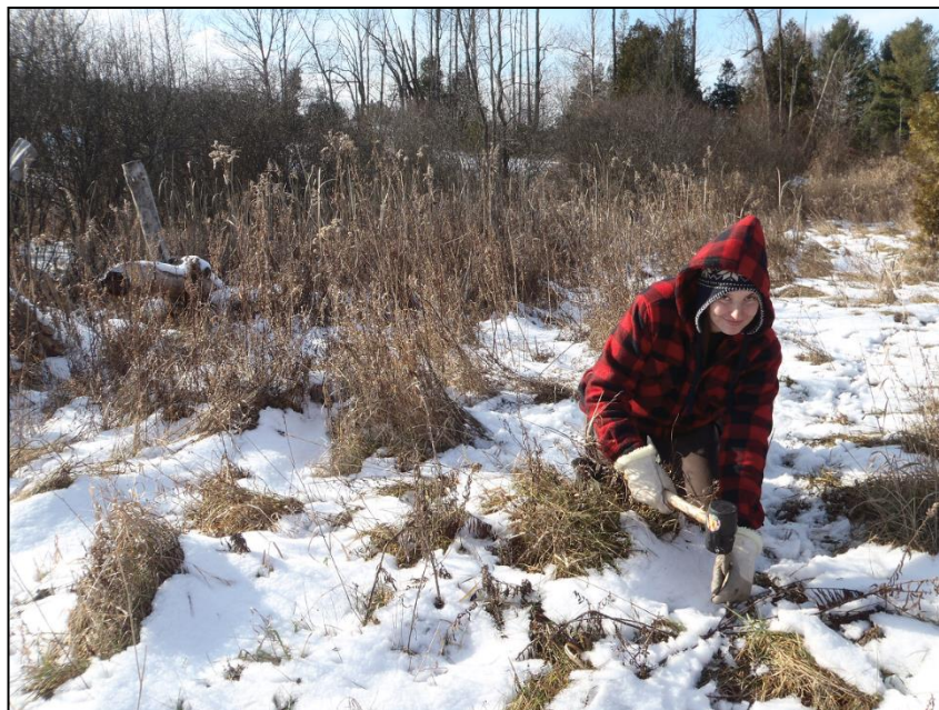
Figure 1: CSSP staff member hammering live willow stake into the wetland.
