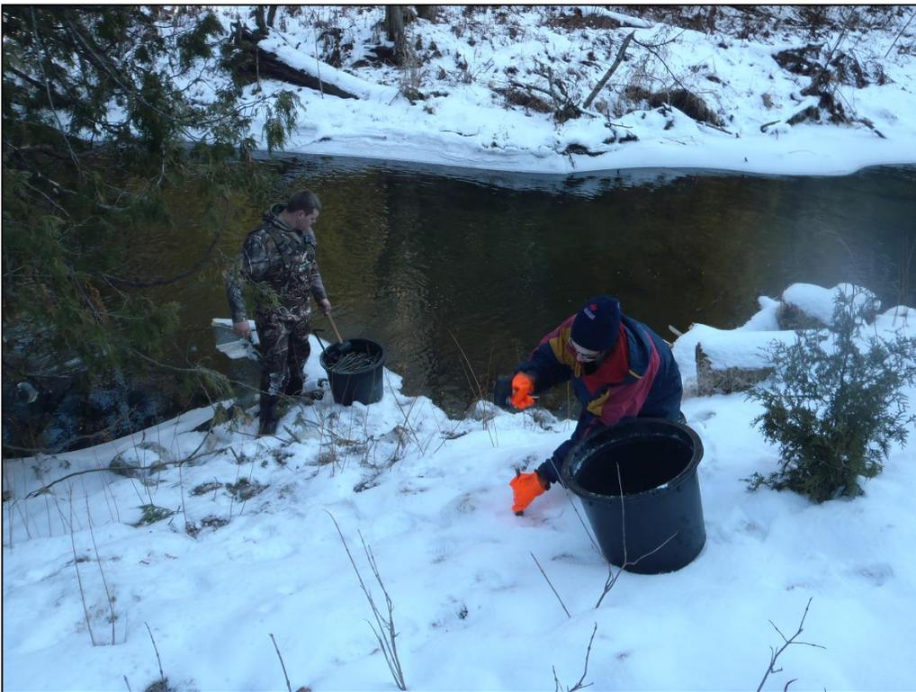
Figure 3: The crew inserting the willow stakes with a mallet.
