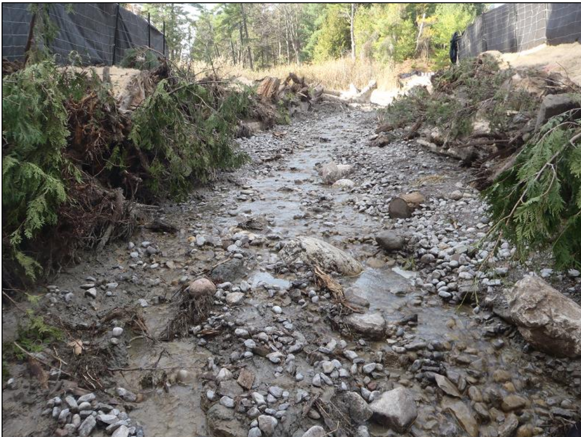
Figure 5: New stream channel.
