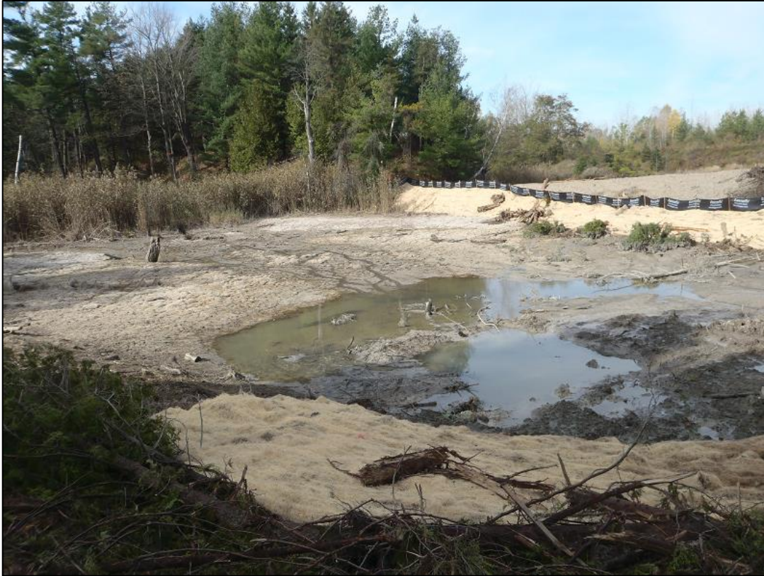
Figure 4: Drained pond and the berm (right) installed to separate the stream from the wetland.
