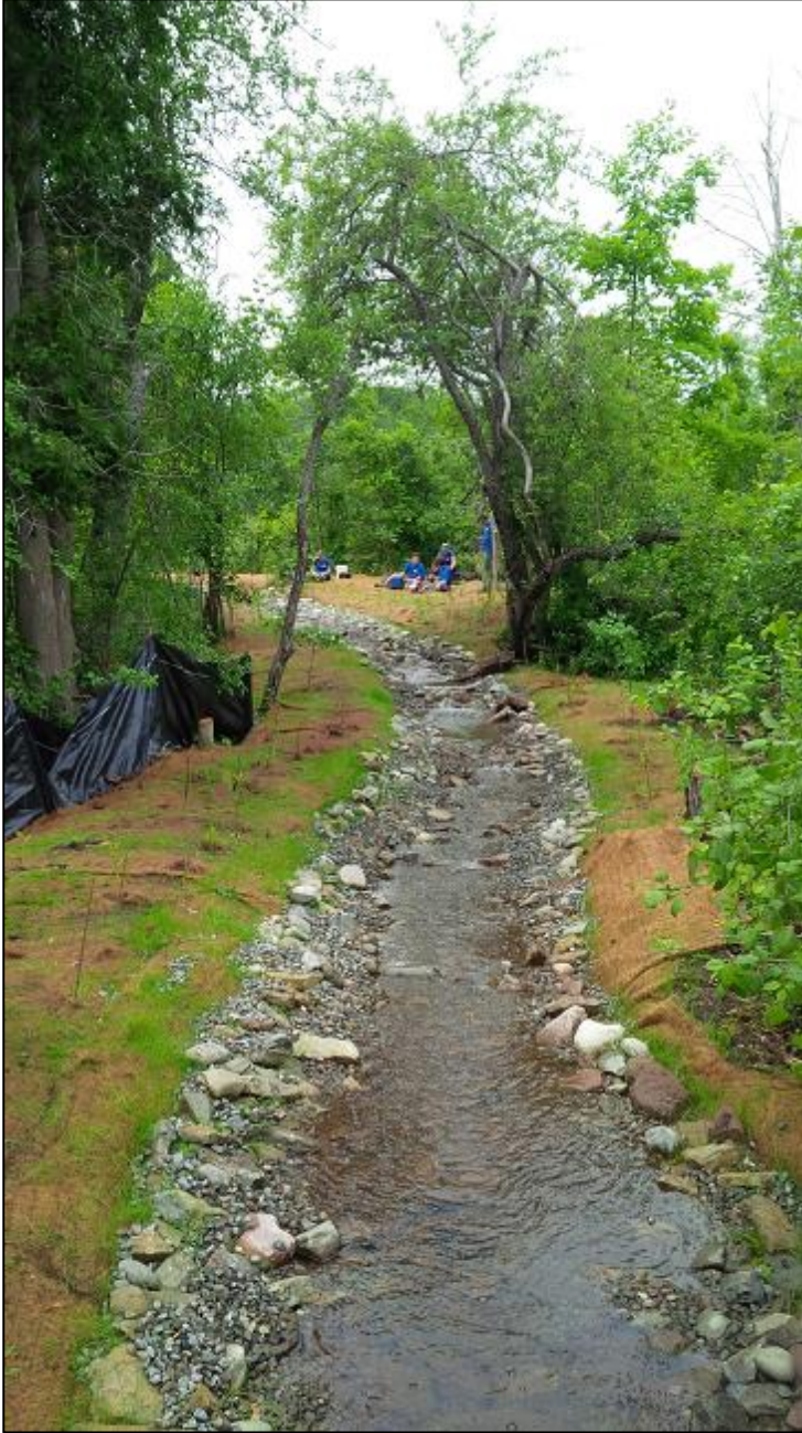
Figure 2: Bypass channel completed with water flowing, photo facing downstream.
