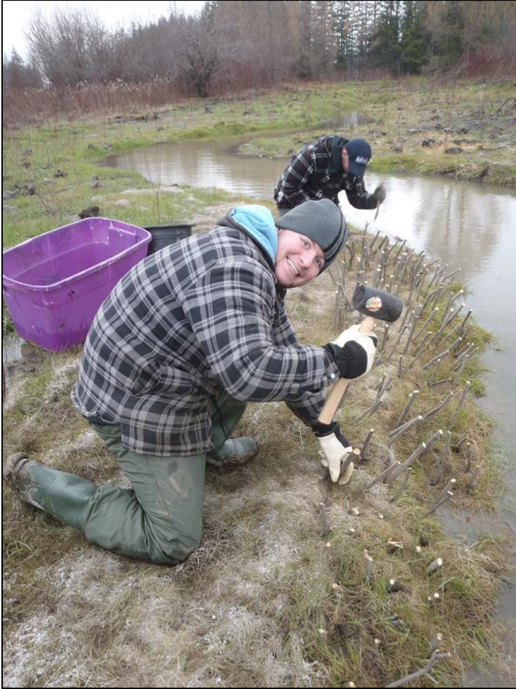
Figure 2: OFAH co-op students installing stakes.
