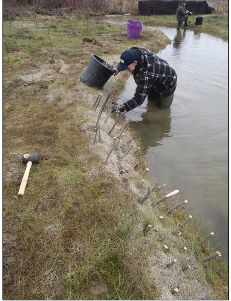
Figure 3: Installing live willow shrub stakes.
