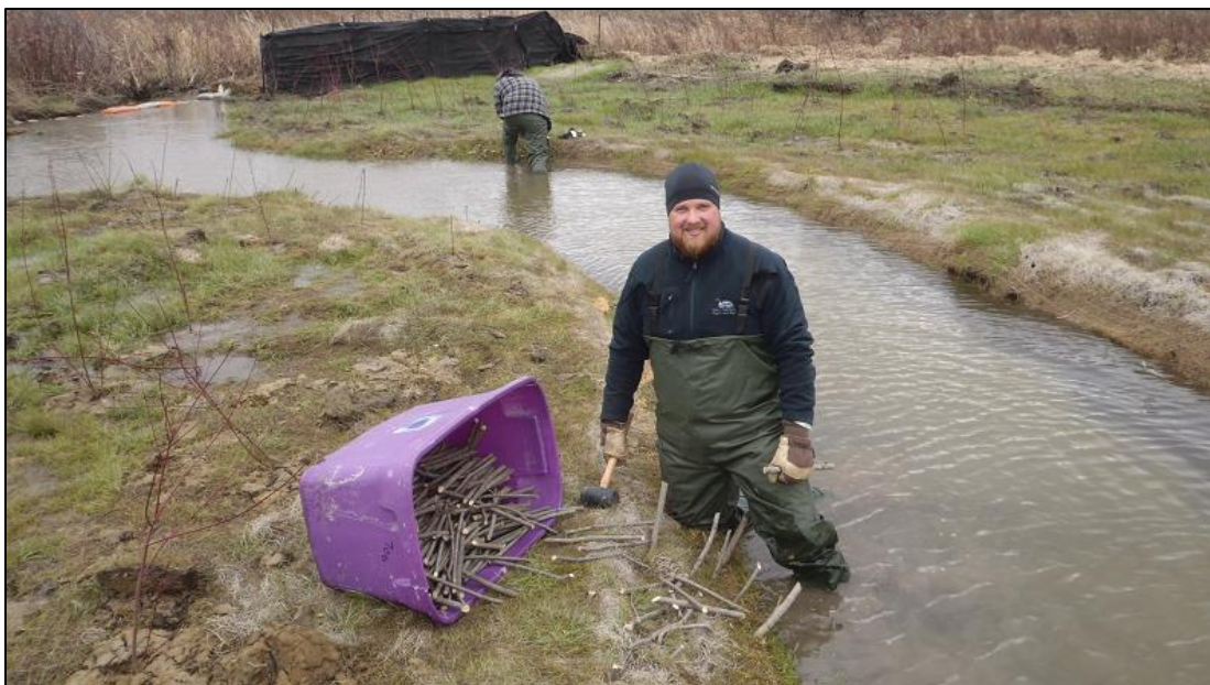
Figure 1: OFAH staff and co-op students installing live willow shrub stakes.
