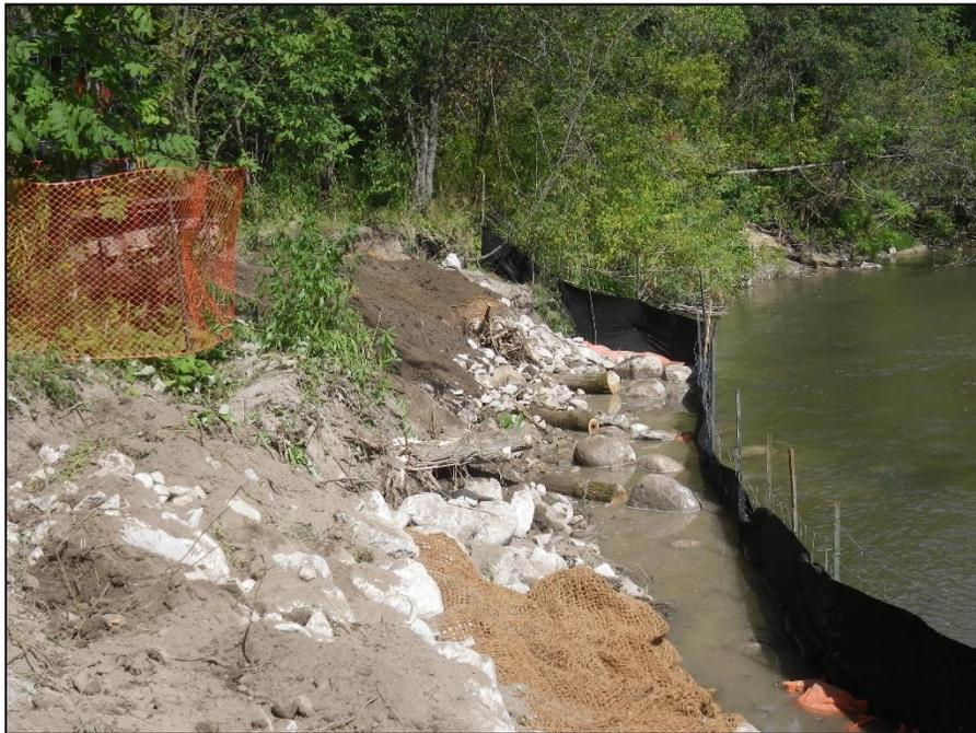
**Figure 2:** Bank stabilization during construction.
